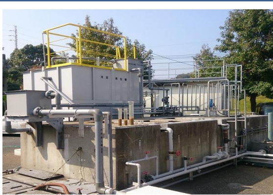
Remodeling. FR*:20ton/day In 2015 (Food processing company)
